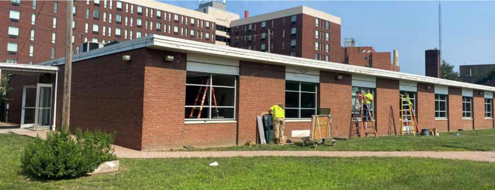
Crews work to install new windows for Mary's Home, replacing the windows that were original to the building.
